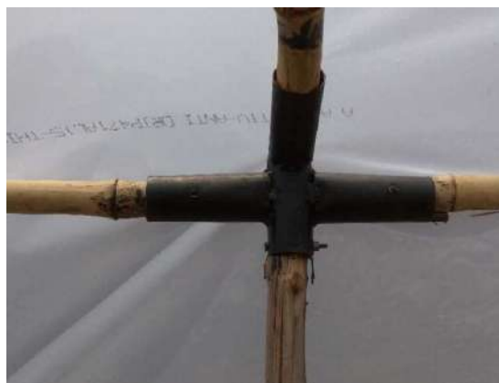
F-13.1.3-D- Bamboos Fitted into MS Pipes with Nut and Bolt Mechanism
